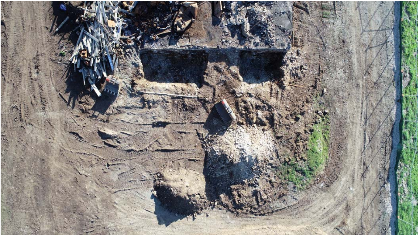
Tank excavations and stockpiled soil on the afternoon of 15 April 2020 following tank removal and soil validation sampling.
