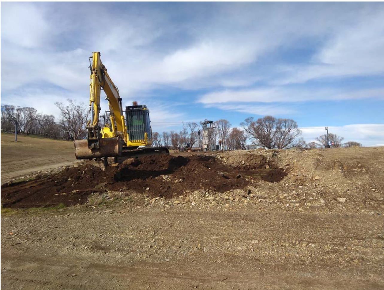
Excavation were backfilled with soil and rock borrowed from the immediate surrounds.
