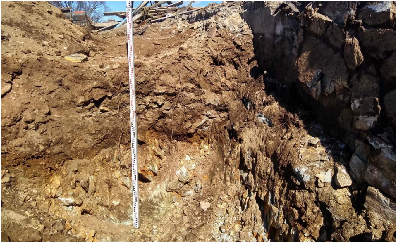
Soil profile on the southern wall of the Tank 1 excavation. Phyllite bedrock was encountered less than 1m below the ground surface.
