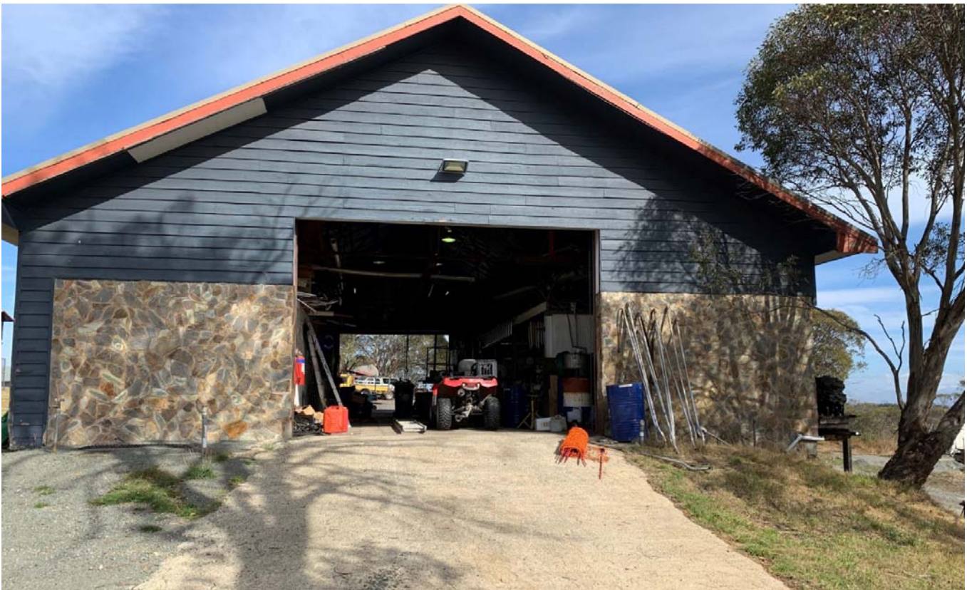
The former Workshop prior to the January 2020 bushfires. Fill pipes and vent pipes are either side of the driveway. Tank 1 on the right side and Tank 2 on the left side.
