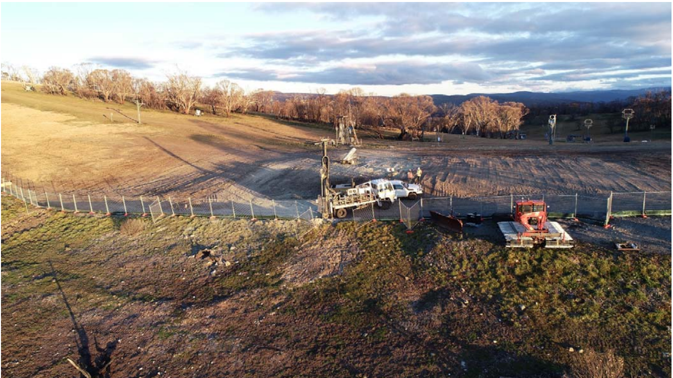
Groundwater monitoring well installation works – 28 May 2020.
