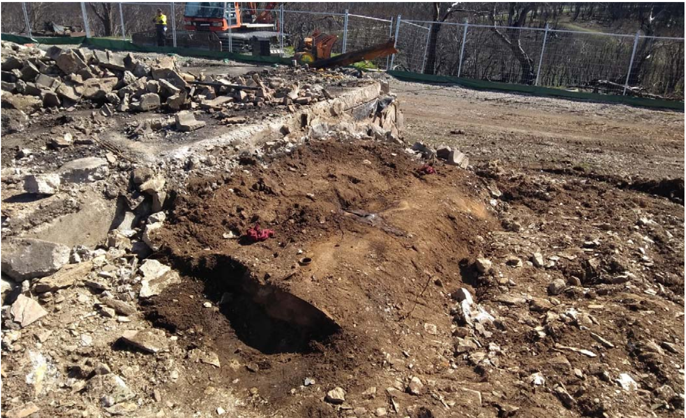
The exposed top of Tank 1 prior to removal.
