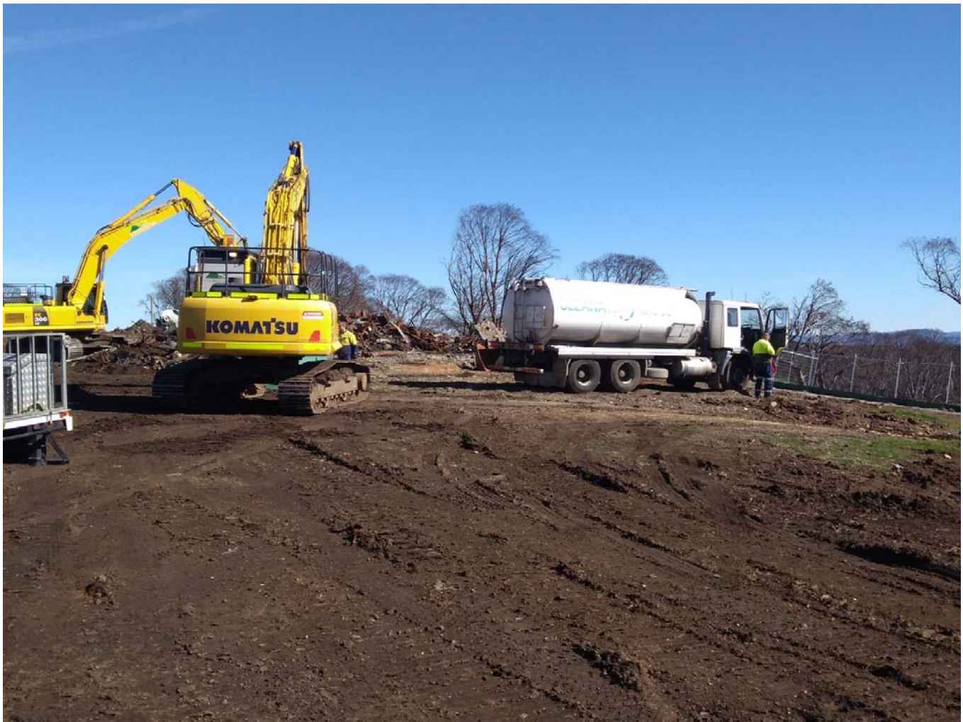
Liquid waste was collected and disposed by Cleanaway prior to tank removal.
