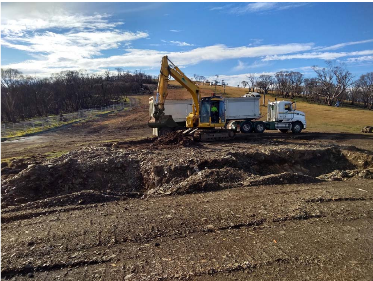
Loading out hydrocarbon impacted soil on 27 May 2020 for off-site disposal.
