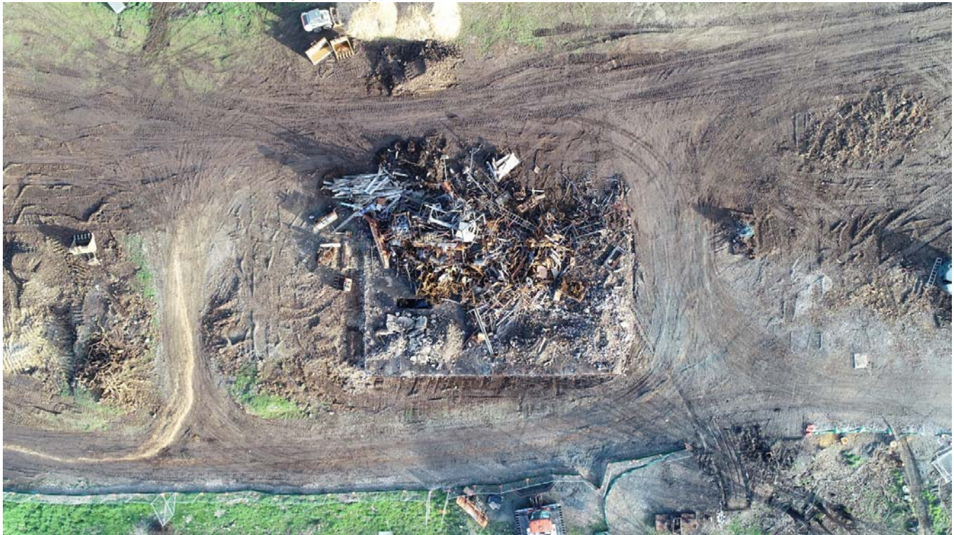
Aerial photo showing the concrete floor of the former workshop. Exposed tops of Tank 1 and Tank 2 are visible on the left hand side of the slab.
